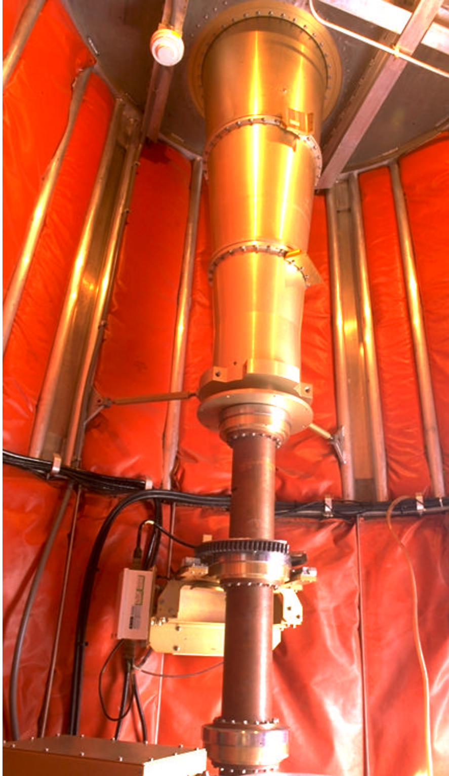
The upper part of the picture is the X-band feed horn. Below is the X-band polarizer. Interesting, huh?
