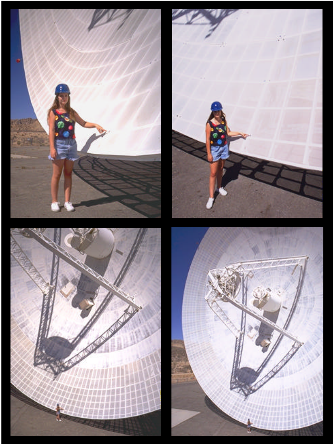
Here I am pointing to one of the dish panel alignment adjusting screws. Notice the camera has moved further and further away for each picture. Can you find me in the pictures above? That dish is huge!
